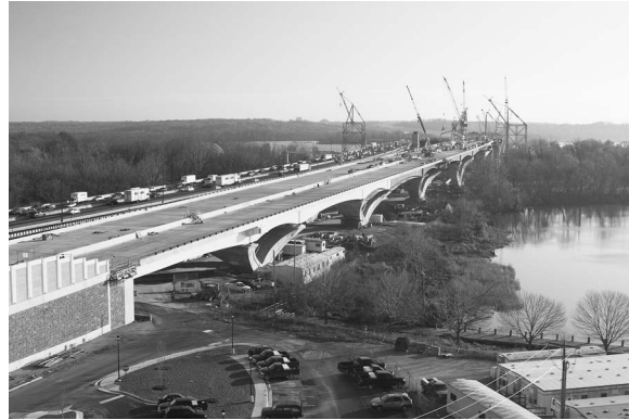
Figure 2. The Virginia Approach Span contract has been a great example of partnering success (© 2005 David Sailors, with permission)
