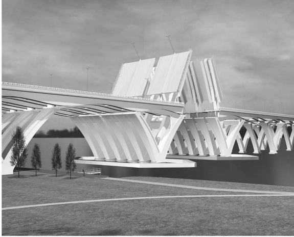
Figure 1. Rendering of the new Woodrow Wilson Bridge; completion is scheduled in 2008
