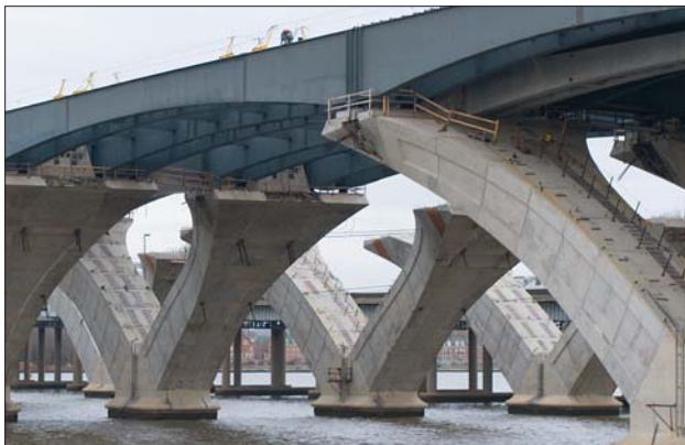
Seen here during construction in late 2005, the new Woodrow Wilson Bridge features an arched V-pier support scheme, reflecting the aesthetics of other nearby Potomac River Crossings. Photo by David Sailors.
