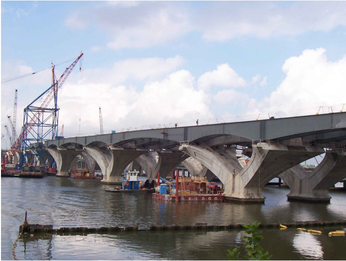
FIGURE 4: Construction of the Woodrow Wilson Memorial Bridge.
