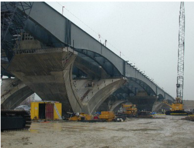
FIGURE 5: Construction of the Virginia Spans Showing Completed V-Piers and Girders
