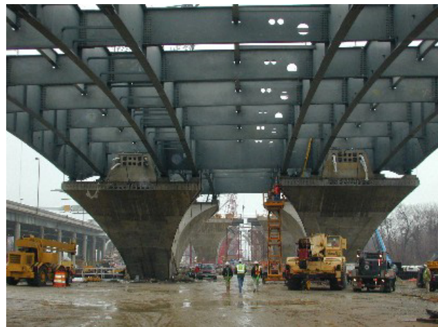
FIGURE 6: Construction of the Virginia Spans Showing Diaphragms and Girders
